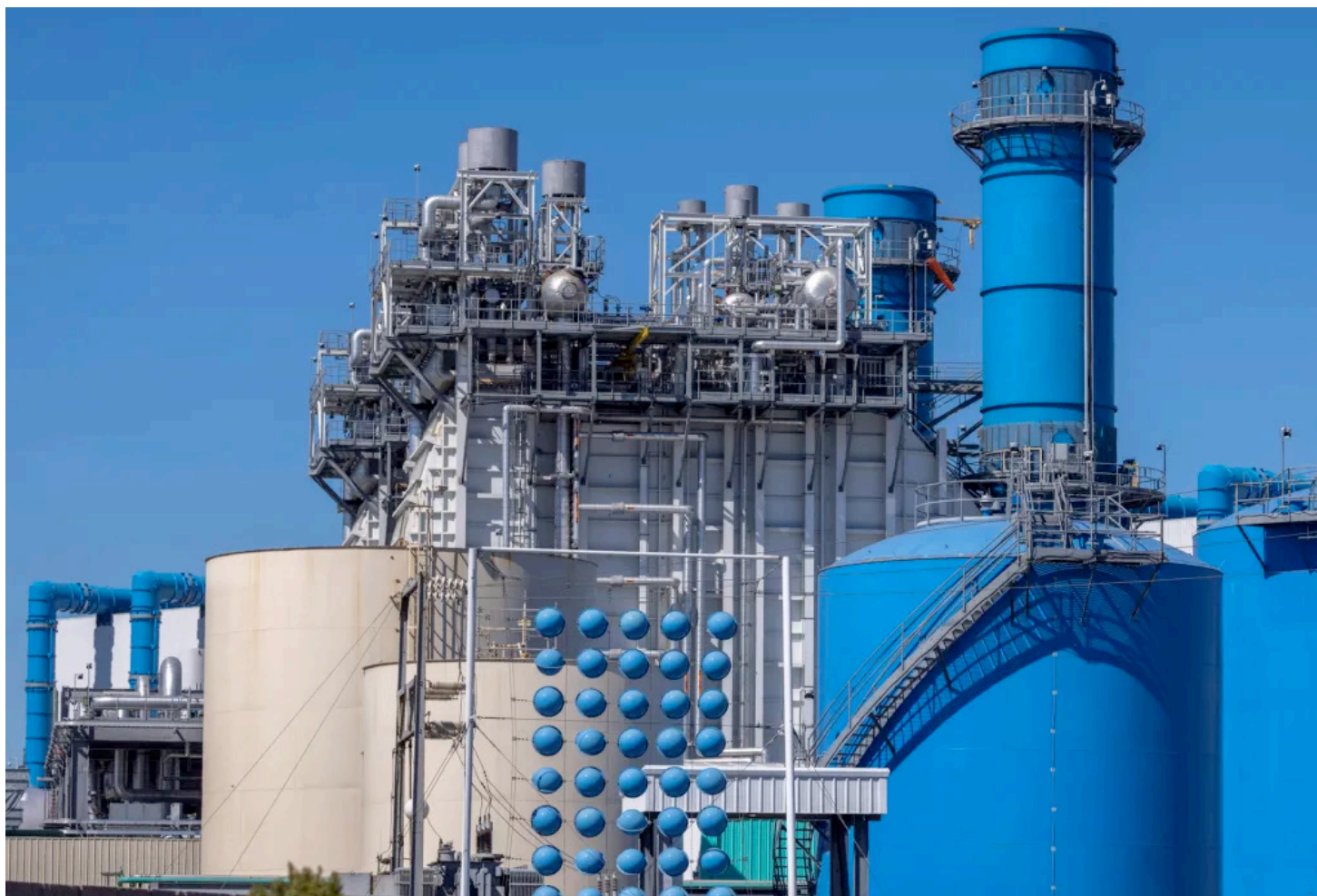
One of California's four natural gas-fired power plants that are set to close next year is in Huntington Beach.
